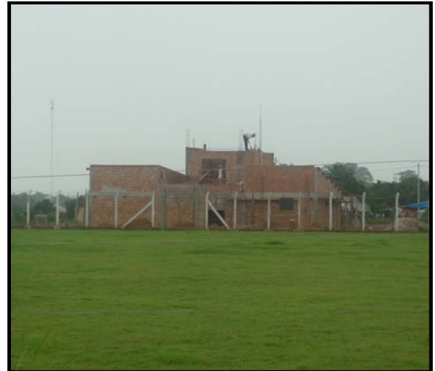
Floresta do Araguaia Football Complex under construction
