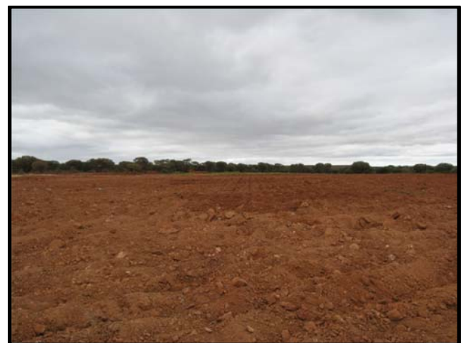
Contractor’s Workshop Infrastructure Area Cleared and Ripped Ready for Seeding
