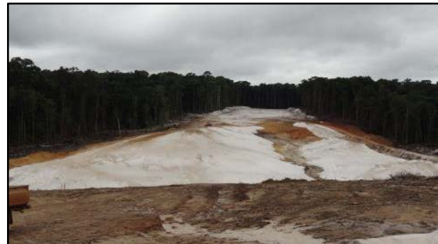
Tailings dam preparation
