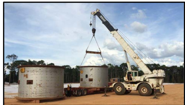
First Stage Plant Construction
